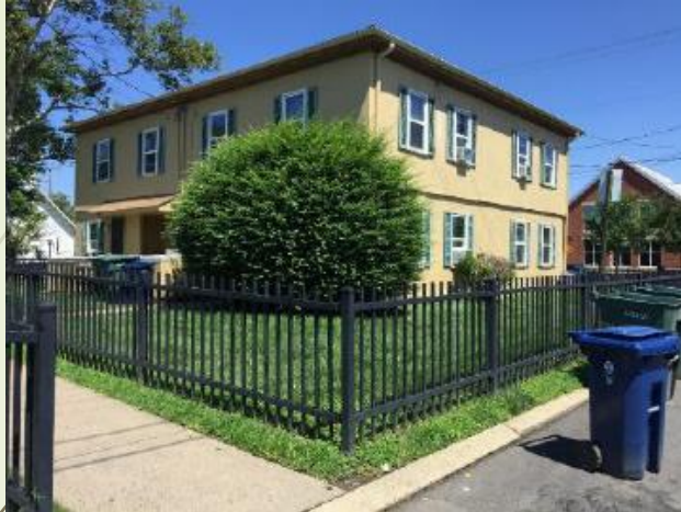
Ramsey Homes, Building I
