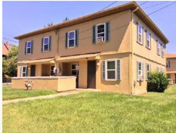
Ramsey Homes, Building IV
