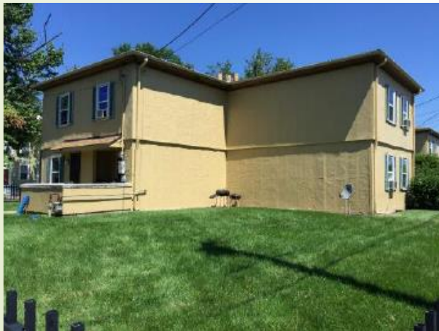
Ramsey Homes, Building II
