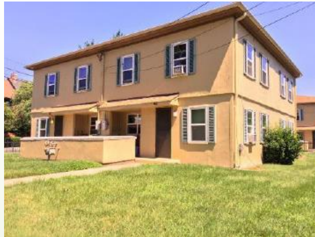
Ramsey Homes, Building IV
