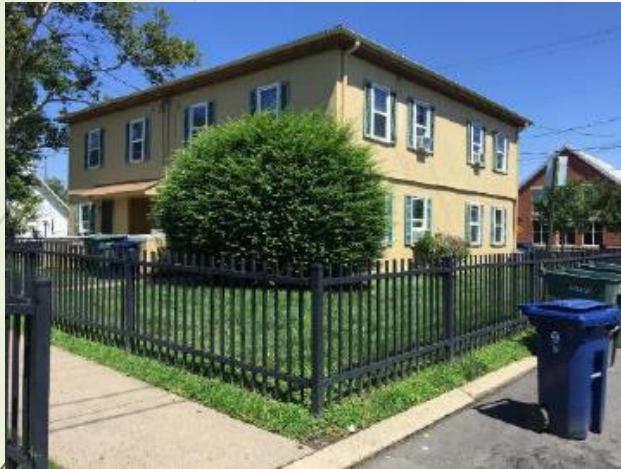
Ramsey Homes, Building I
